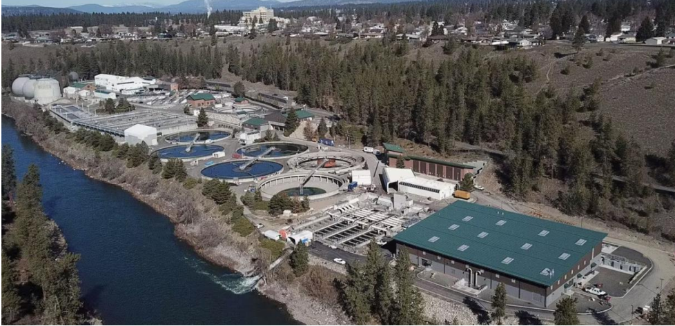
Figure 1. Spokane's Riverside Park Water Treatment Plant (Water Management, 2024)
